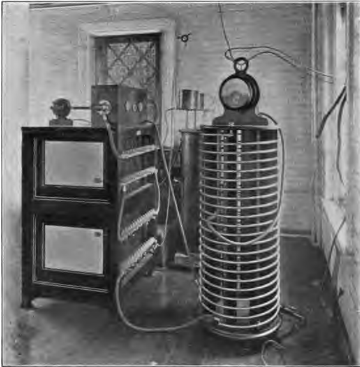
FIG. 8. — HIGH-POWER OUTFIT, WITH ROTATING SPARK-GAP MOUNTED ON LEYDEN-JAR BATTERY FRAME, AND HOT-WIRE CURRENT METER MOUNTED ON INDUCTANCE FRAME. —Navy Yard, Washington, D. C.
